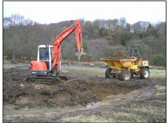
Pond Creation as part of mitigation works ©Gateshead Council
