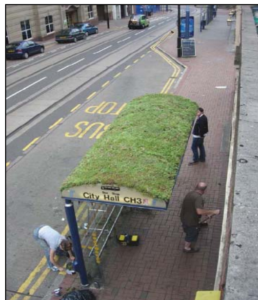
Green Roof on a bus shelter ©The Green Roof Centre
